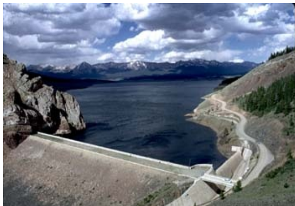
Taylor Park Dam and Reservoir - USBR photo
