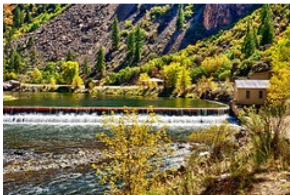
East Portal of the Gunnison Tunnel
