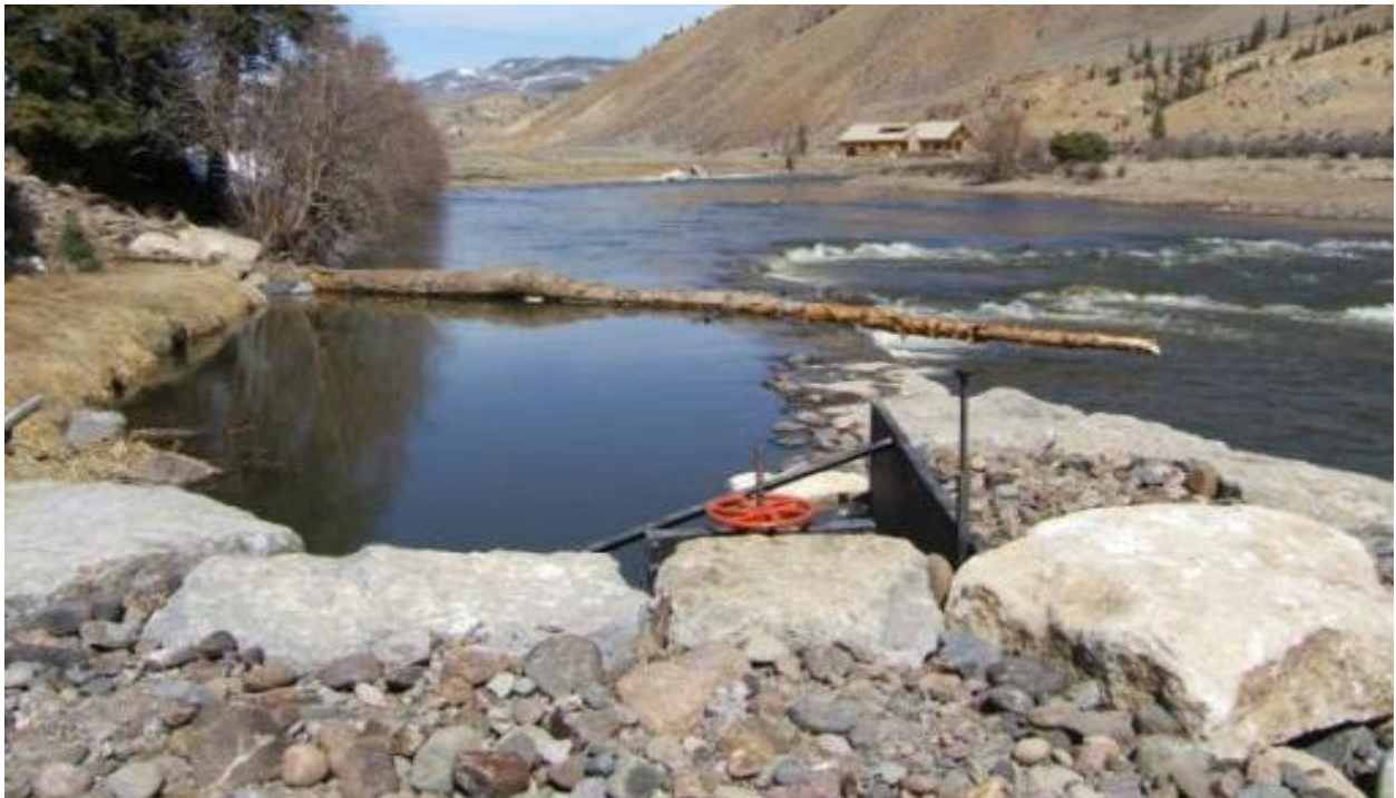
Photograph 20. Photograph of engineered diversion structure provided by Elk River Construction, Pagosa Springs, CO.
