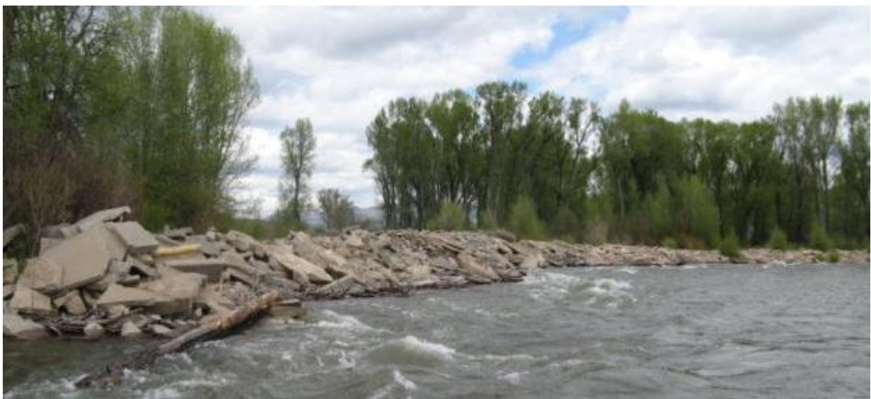
Photograph 16. Photograph taken during peak runoff, 2010, of bank armoring of the Gunnison River (Gunnison County, CO) upstream of the confluence with Ohio Creek near Van Tuyl Ranch.
