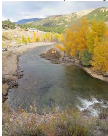
Figure 5. Reshaping of the flood plain and structure installation below the 8 ½ Street Bridge (fall 2016). The second to last photo is looking back toward the bridge and shows where a large area of berm was removed (compare to pre-construction photo Figure 3, second photo). Last photo is the area after one year of high flow (fall 2017).
