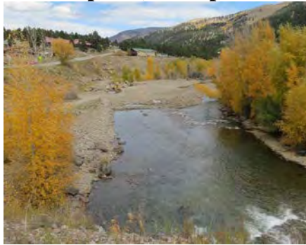
Figure 5. Reshaping of the flood plain and structure installation below the 8 ½ Street Bridge (fall 2016). The second to last photo is looking back toward the bridge and shows where a large area of berm was removed (compare to pre-construction photo Figure 3, second photo). Last photo is the area after one year of high flow (fall 2017).
