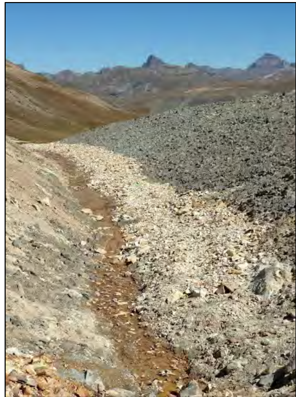
Photo 8-3: Drainage from the Hough Mine en route to North Palmetto Gulch in September 2016, one year following reclamation. The right side of the photo includes edge of the mine waste repository.
