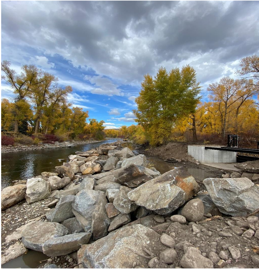
It is almost complete! Some minor channel work will wrap up the project soon.
