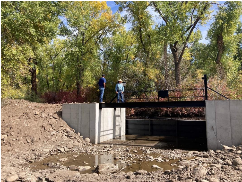
The new diversion structure was engineered specifically for the project.
