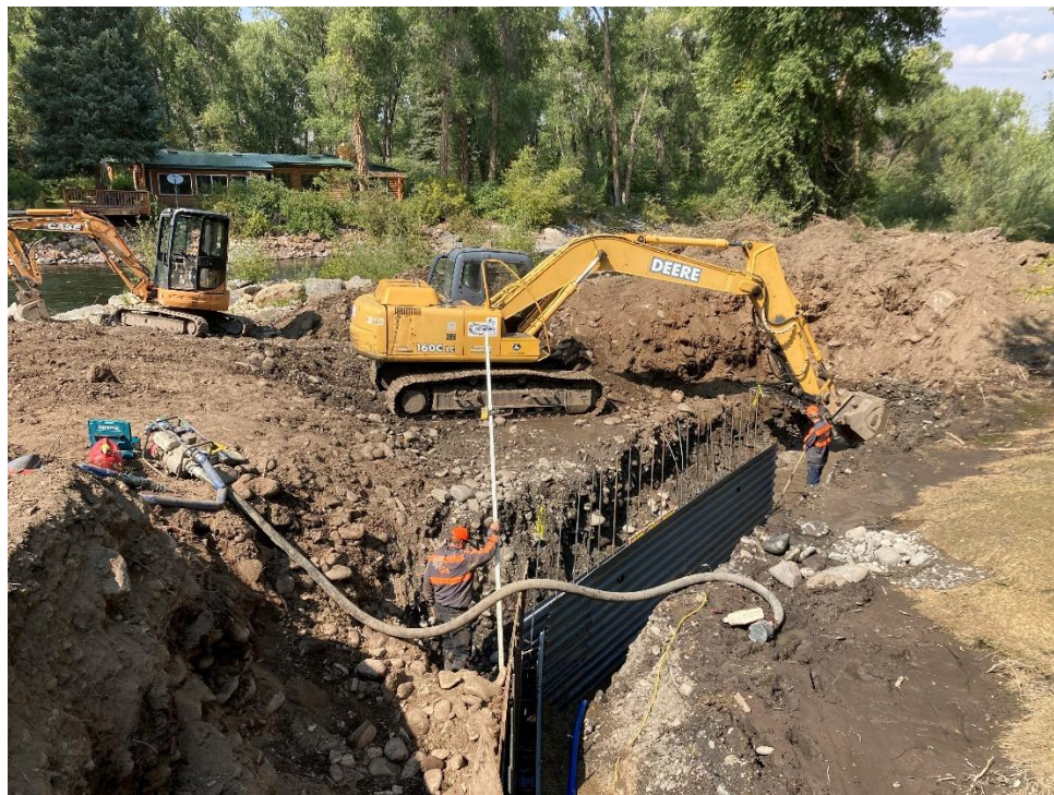
Using heavy machinery, trenches are dug in preparation for pouring footers.
