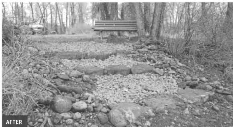
The restoration project created cobble ramps and pathways that will help prevent erosion and encourage vegetation to grow back along the river bank.
