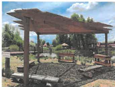
Permanent shade structure. Additional work tables and benches for classes of students still to come.
