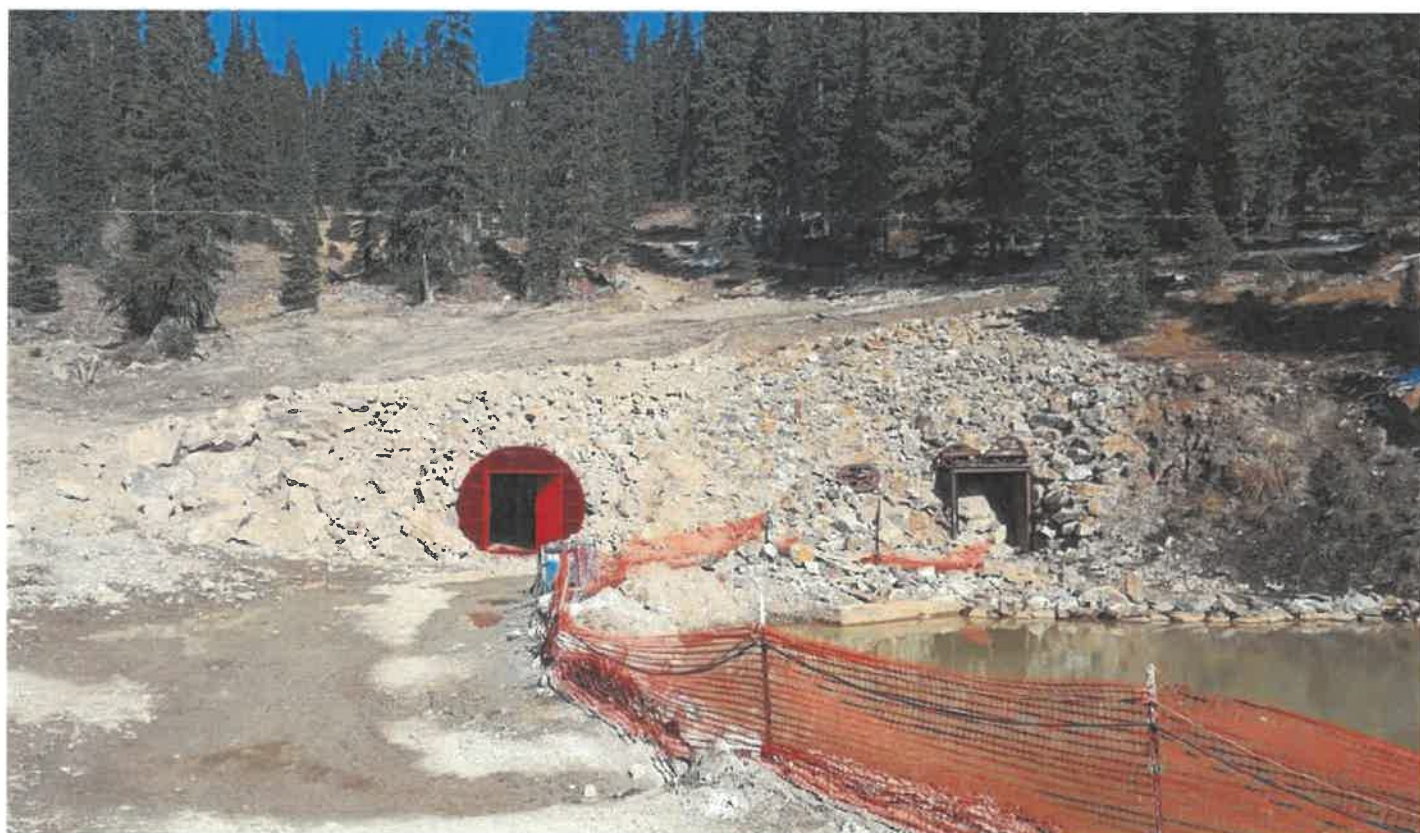
Level 1 bypass adit (red door) and original Level 1 adit at Standard Mine | EPA
