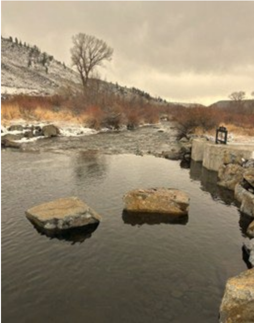
Chittenden Ditch Diversion
