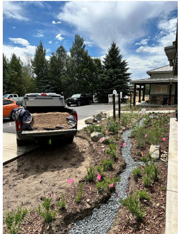
Photo 8: Planter adjacent to office building. Rose granite installation.
