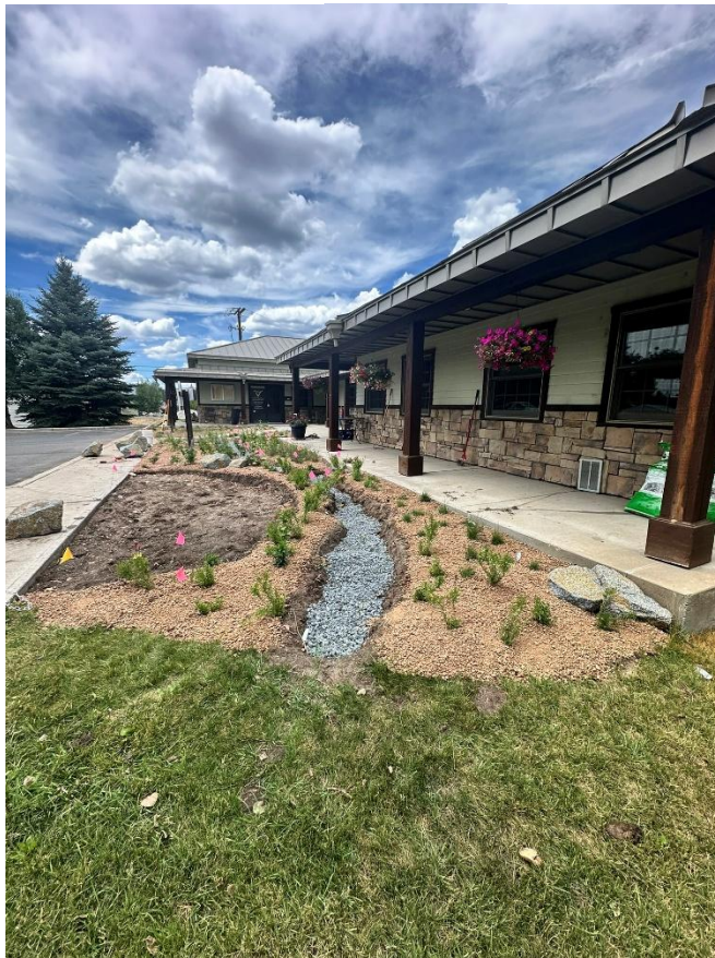
Photo 12: Planter adjacent to office building after rose granite installation.
