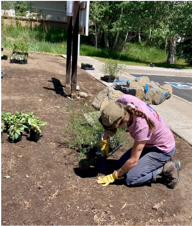
Photo 5: Amanda Aulenbach installing plants.
