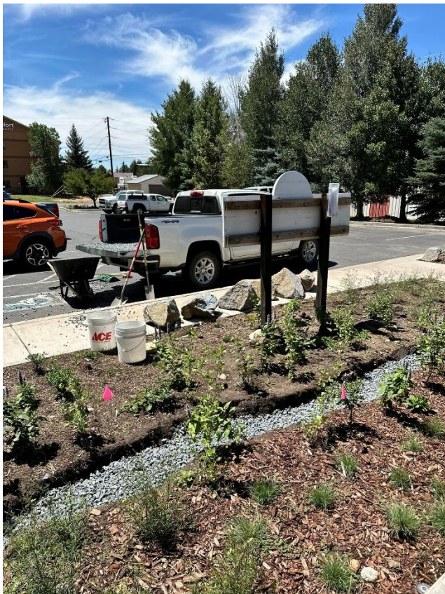
Photo 9: Planter adjacent to office building during blue granite "river-scape" installation.
