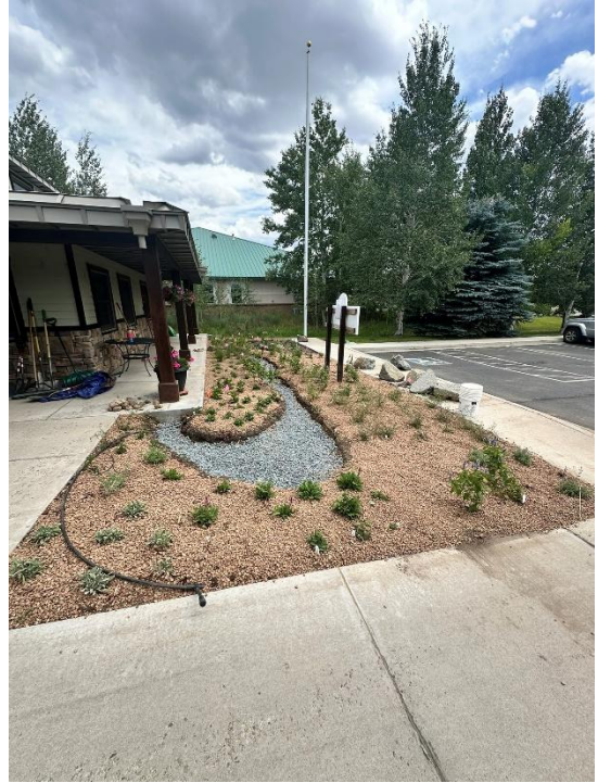
Photo 10: Planter adjacent to office building after rose granite installation.
