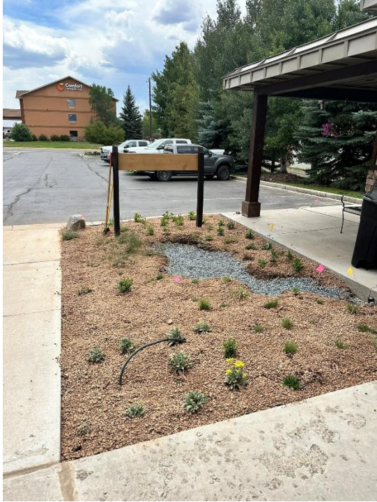
Photo 11: Planter adjacent to office building after rose granite installation.
