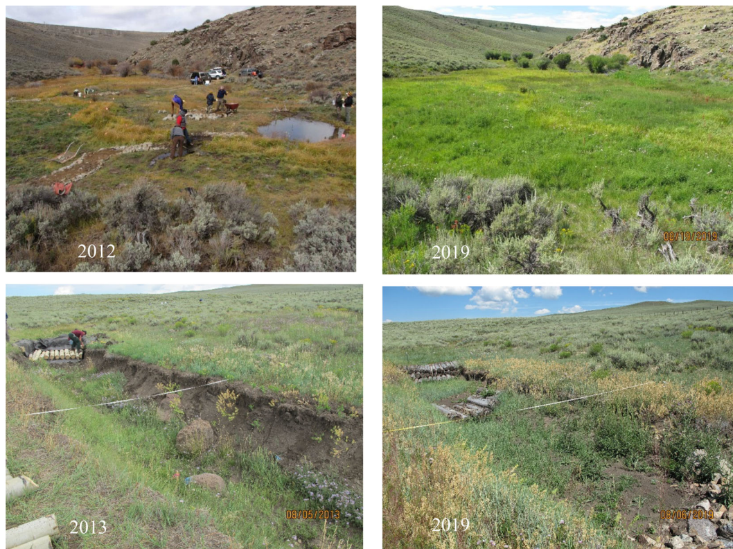
Figure 3. Repeat photos demonstrate the increase in wetland cover associated with a media luna structure (top row). The lower row demonstrates a log and fabric structure used to heal a head cut. Note that an additional log structure was added after the 2013 photo was taken. The white ribbon visible in the lower photos marks one vegetation transect; note the depth of the stream incision and sediment build up below the tape in both photos. All photos were taken within a few Julian weeks of the original photo.
